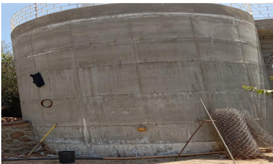
Figure 15: Concrete water tank constructed by MoEWA, Shada Al Baha
